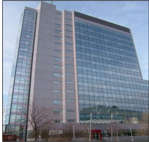
The new Kosovo Government Building, completed in early 2006, now houses the ISSR Secretariat alongside the OPS.
